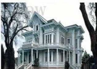
Standalone Access Control House
