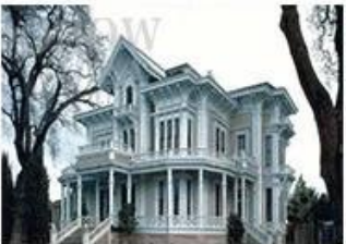
Standalone Access Controt House
